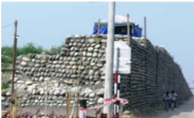
Figure 5. Unfinished cobble and concrete gravity retaining structure in Hanwang, Sichuan Province, China, following the 5-12 Sichuan Earthquake.
